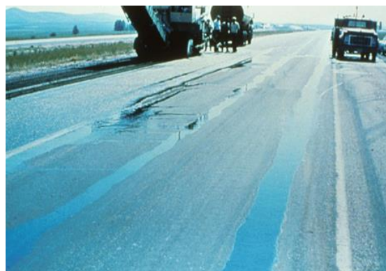
Figure 6: Examples of rutting distress in asphalt pavement.
