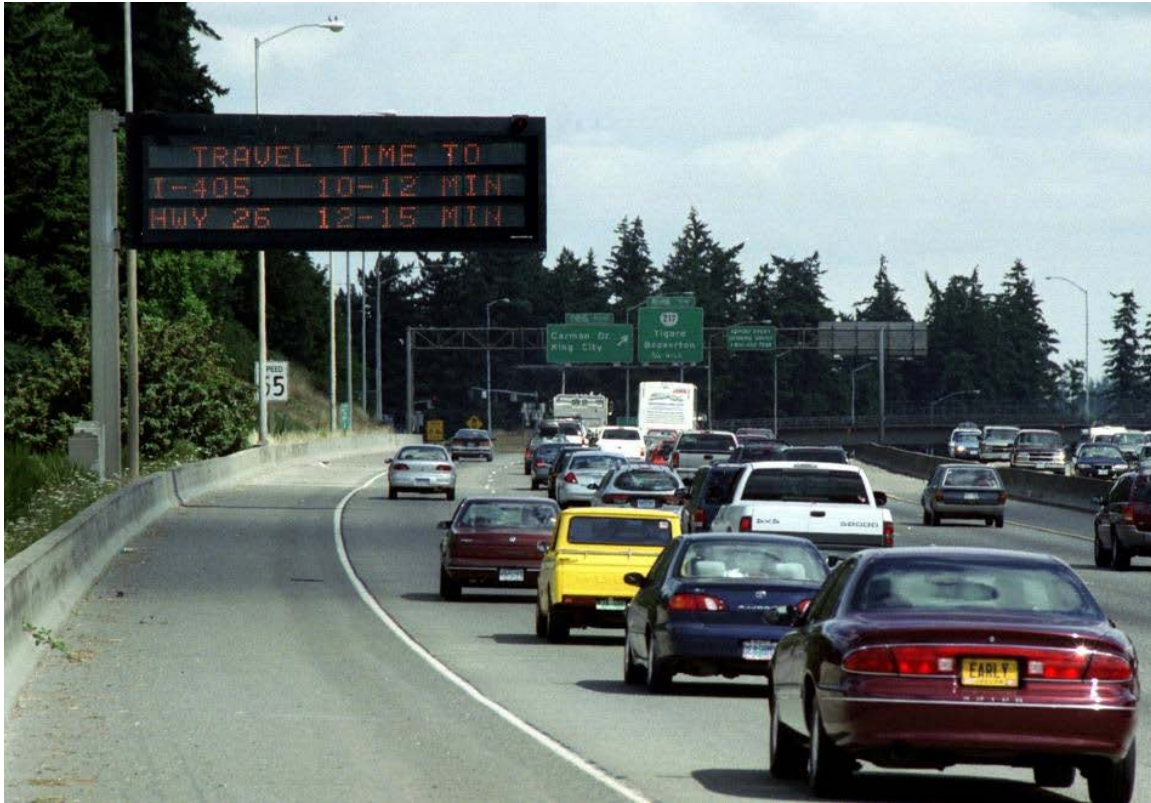
An example of a dynamic message sign time window in Oregon. ( http://otrec.us/news/entry/report_travel_time_data_lacking_at_key_spots_on_portland_area_freeways )
